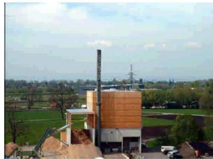
Guardbridge Biomass district heating
